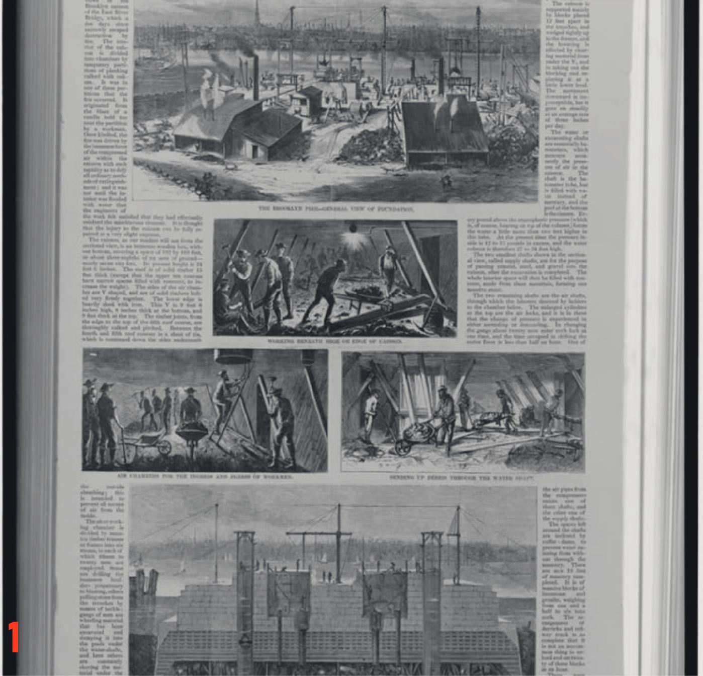
Plate 1 — Falsework: the timber frame of the East River caisson, built in order to be destroyed or buried. Harper's Weekly, 1870.
