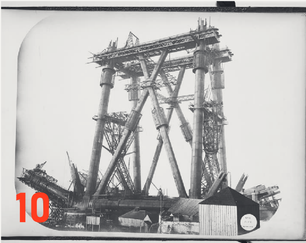
Plate 10 — The Forth cantilevers: self-supporting at every stage, because no centring could be built in that estuary.
