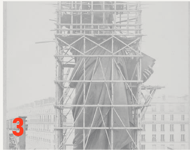
Plate 3 — Paris, 1882: the copper skin rising, plate by plate, on Eiffel's iron armature.
