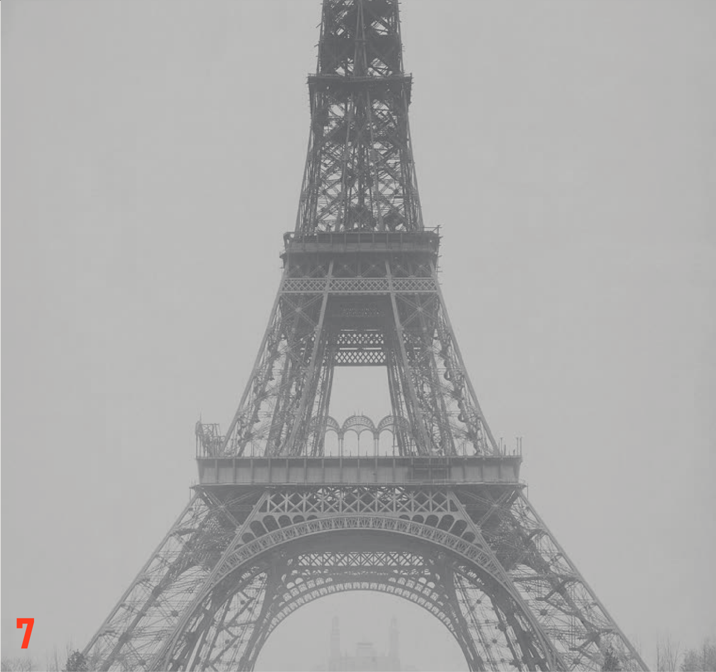
Plate 7 — The tower rising: a scaffold that carries only itself. Louis-Émile Durandelle, 1888.
