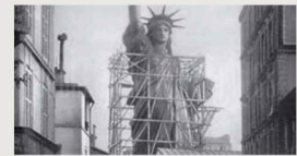
Plate 5 — Falsework and figure, indistinguishable at this hour. construction: two shells, one inside the other, tied by ribs, and between the ribs a herringbone brickwork in which each fresh course was pitched
