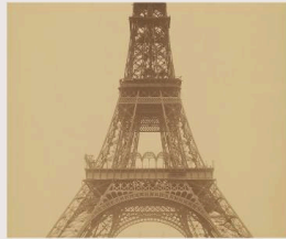
Plate 7 — The lower rising: a scaffold that carries only itself. Louis-Émile Durandelle, 1888
