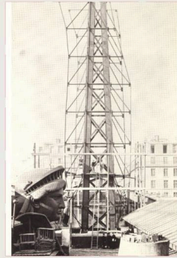
Plate 4 — The statue under assembly. The scaffold outside will go; the skeleton inside will not.
