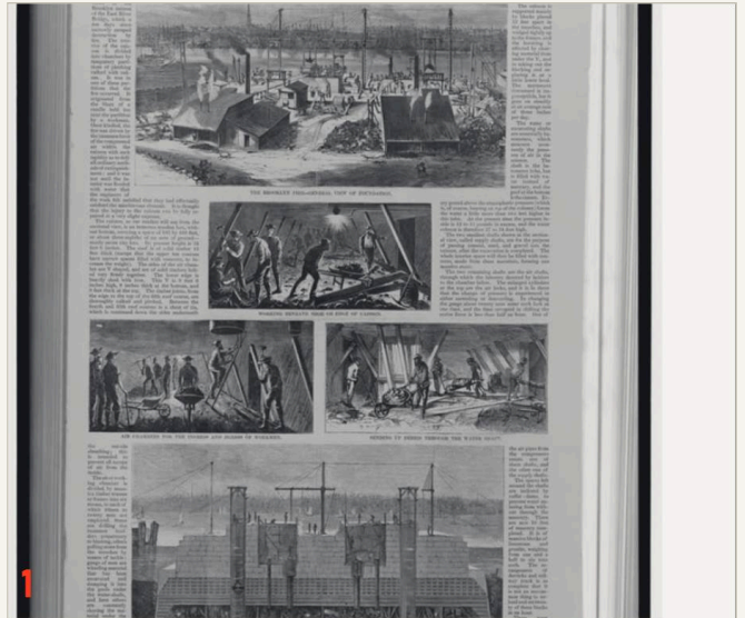
Plate 1 — Falsework: the timber frame of the East River caisson, built in order to be destroyed or buried. Harper's Weekly, 1870.
